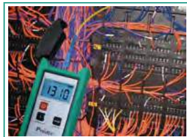
Fiber optic power test
