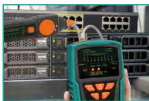
PoE switches & wire tracing
