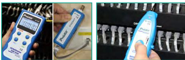
PoE switches & wire tracing
