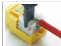
Punch and cut cable terminals
