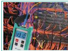
Fiber optic power test
