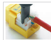
Punch and cut cable terminals
