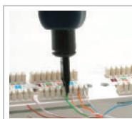
Punch and cut cable terminals
